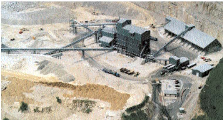
LEFT: An installation for Tarmac in Swindon in 2000
