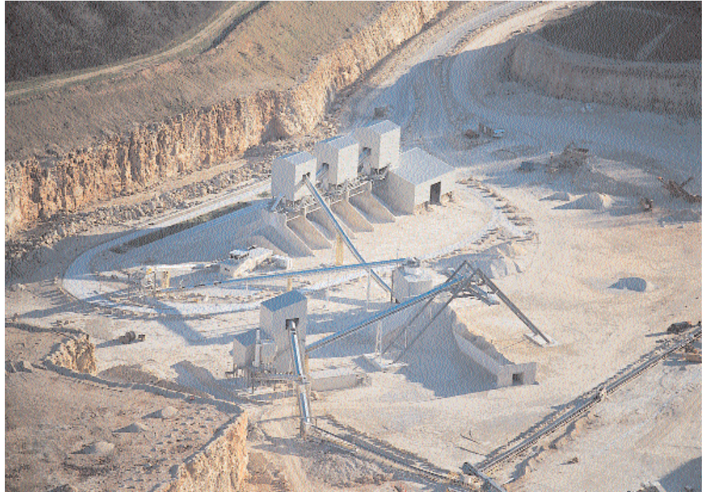
ABOVE: Fairport installed new screening plant at Holme Hall crushing and screening plant in 2004
